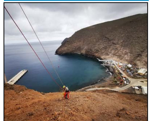
Removing loose rocks above Rupert's Wharf Access Road
