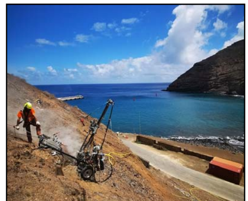
Drilling anchors above Rupert's Wharf Access Road
