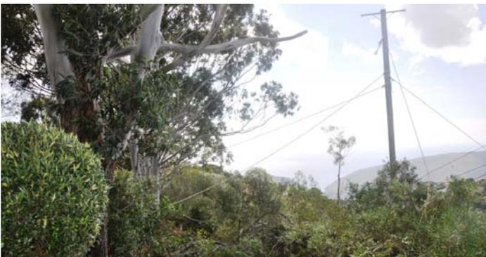
**The new pole is pulled into position. The lower branches of a tall eucalyptus tree were cut back to keep them clear of the power line.**
