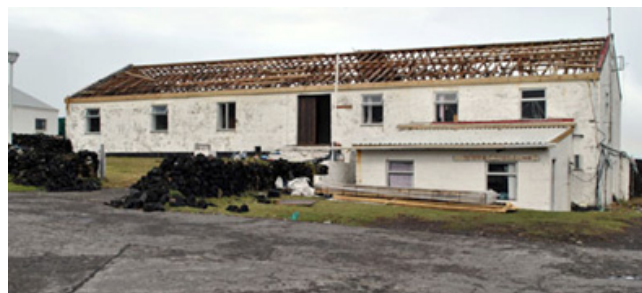
The recently laid roof of the Administation Building was (almost) completely ripped away by the storm overnight on 2nd/3rd November.
