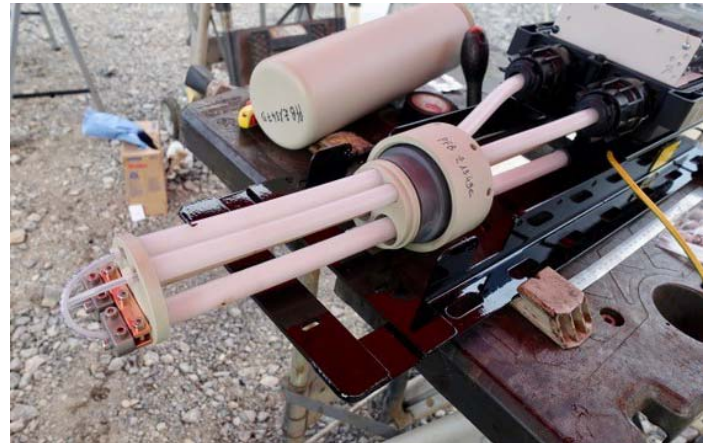
Fibres from land and sea cables in splicing tray enter at opposite sides ready for splicing
