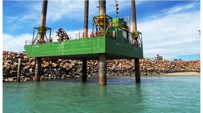
A jack-up barge with a ramp from the seafront will give access to new parking areas
