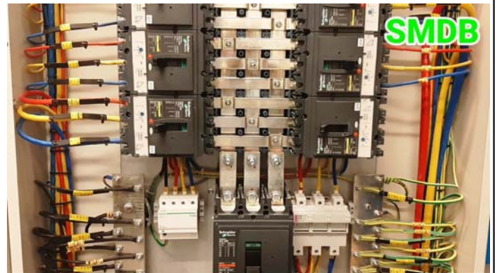
An electrical busbar installation – not necessarily of the same type/design used at the power station
