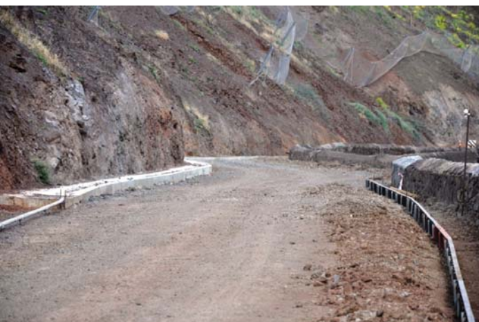
The slipper drain (left) and ducting (right) were laid before the main road surface
