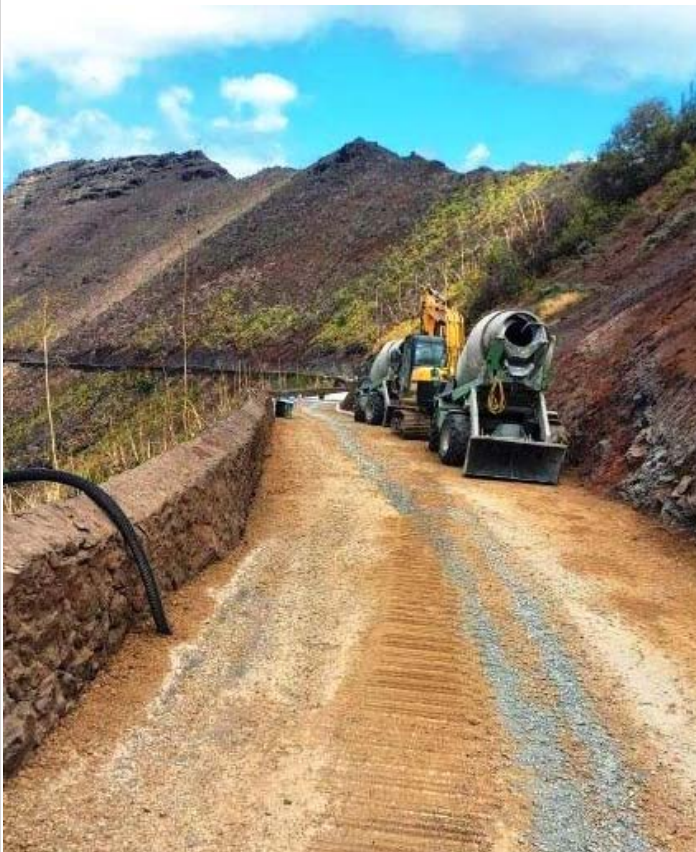
Compaction of the road base before the concrete surface is laid
