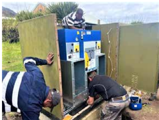
One of the five new Tristan substations is assembled.
