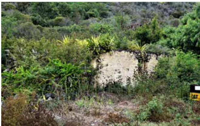
The first stage in restoration was to clear the vegetation to do a detailed survey of what was left of the structure
