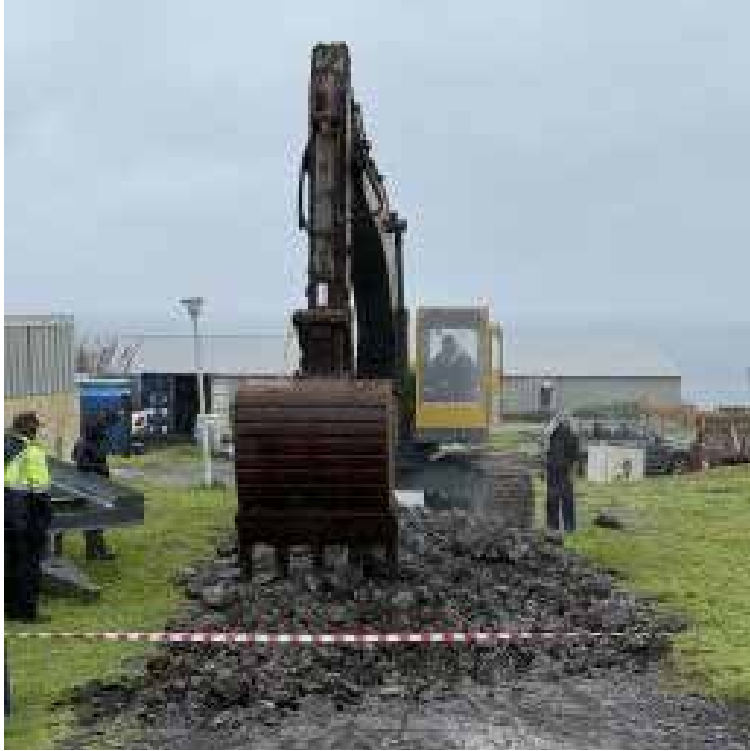
Digging up the old, damaged road surface.
