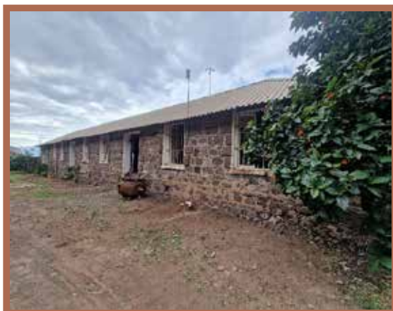
Figure 1- No.1 Building in Rupert's Valley
